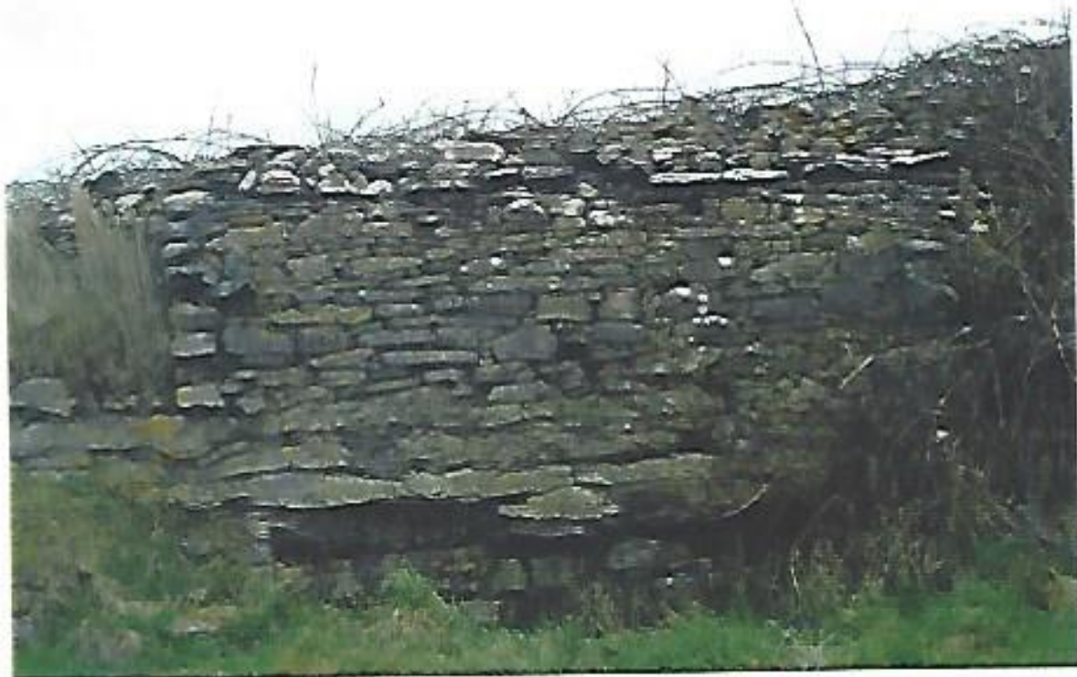
Pl. 13 Looking East at possible building (SL010-01803)
