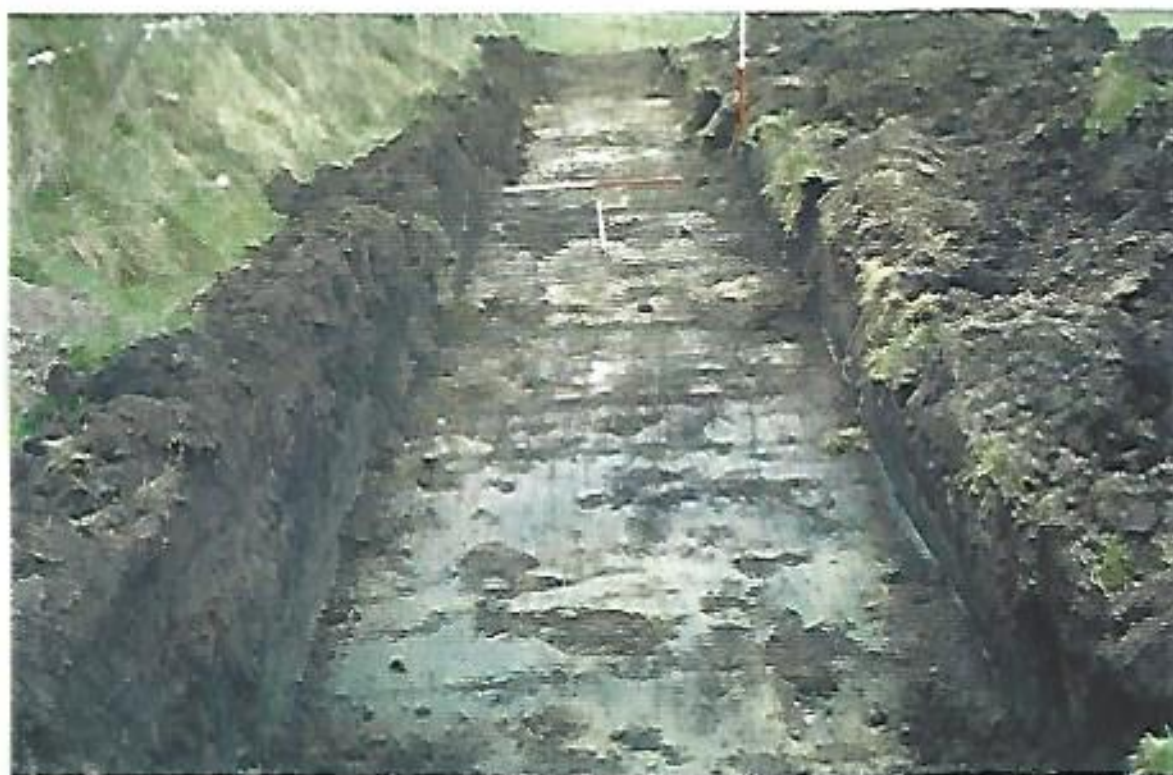
Pl. 9 Looking West along Trench No. 9
